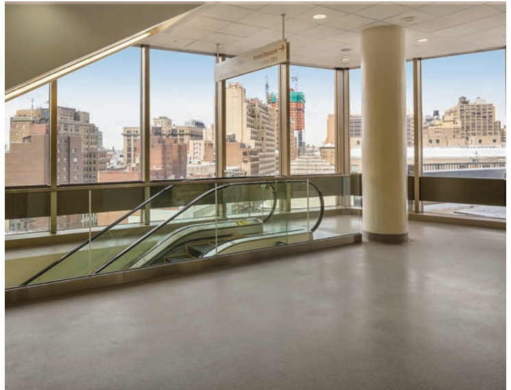
Stonshield SLT was specified for the escalator towers due to its durability, slip resistant texture and decorative appearance
